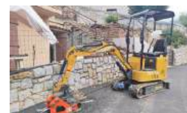
Our excavator in Paris, France.
