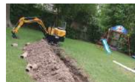
Our excavator in Vancouver, Canada.
