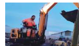
Our excavator in Chile.
